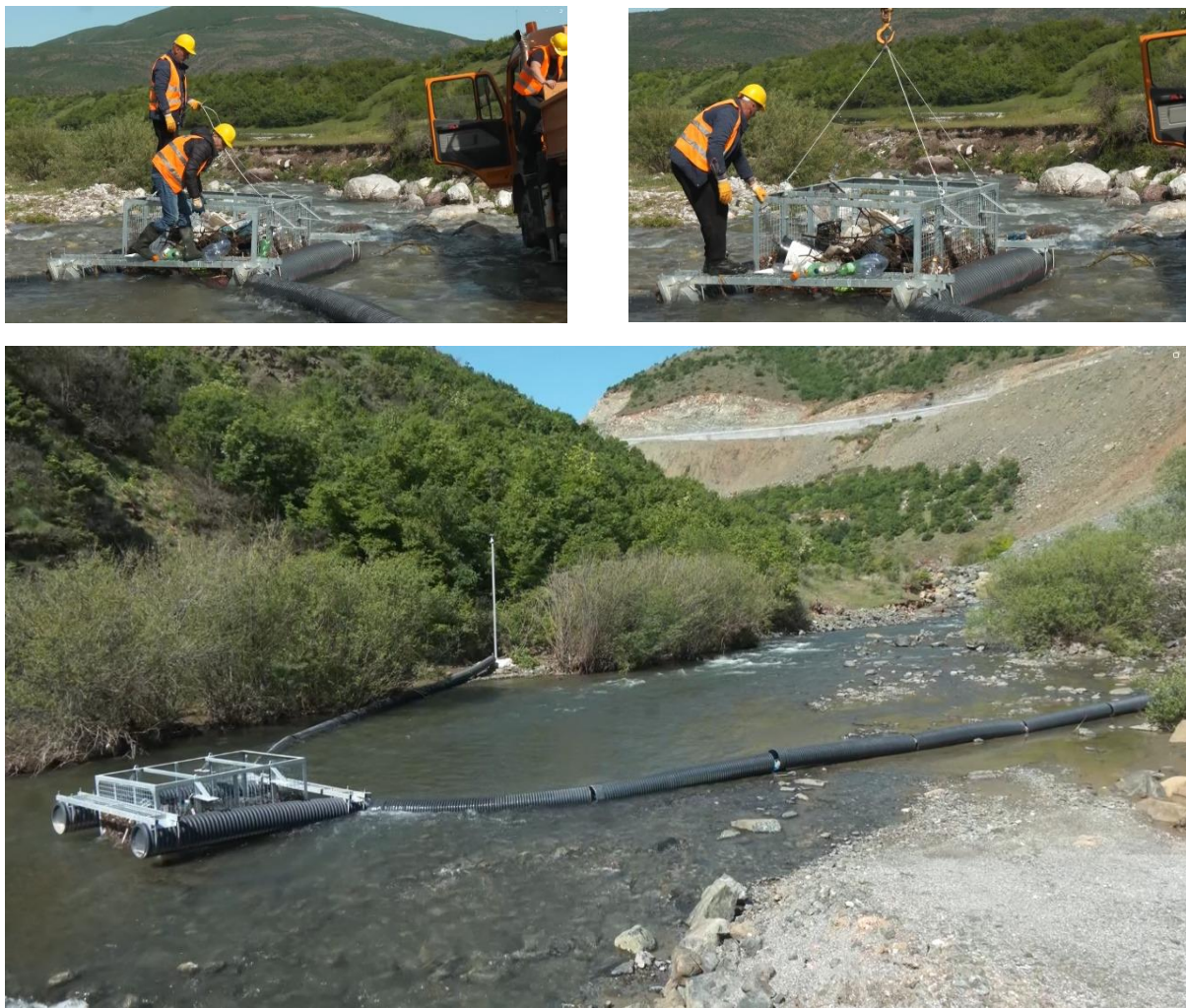
Figure 4: Photo from the positioning of litter traps in water streams in Drini River
